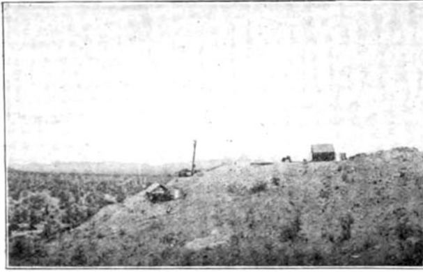
PLOMOSA MILL AND POWER PLANT.
