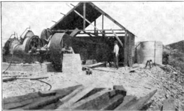
125-HP. LIDGERWOOD HOIST BEING INSTALLED.
