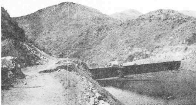
Rare 65-year-old photograph shows the Hassayampa Dam as it appeared during its brief life. View is downstream.
